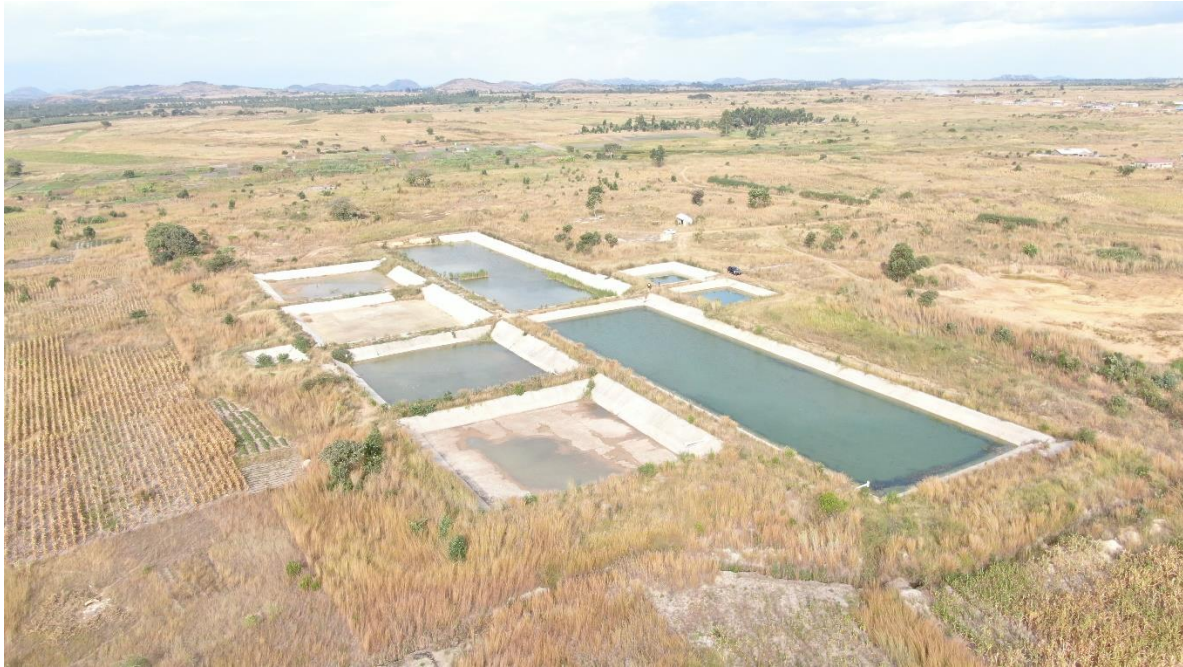
Plate 4.2: Newly Constructed Sewer Ponds
