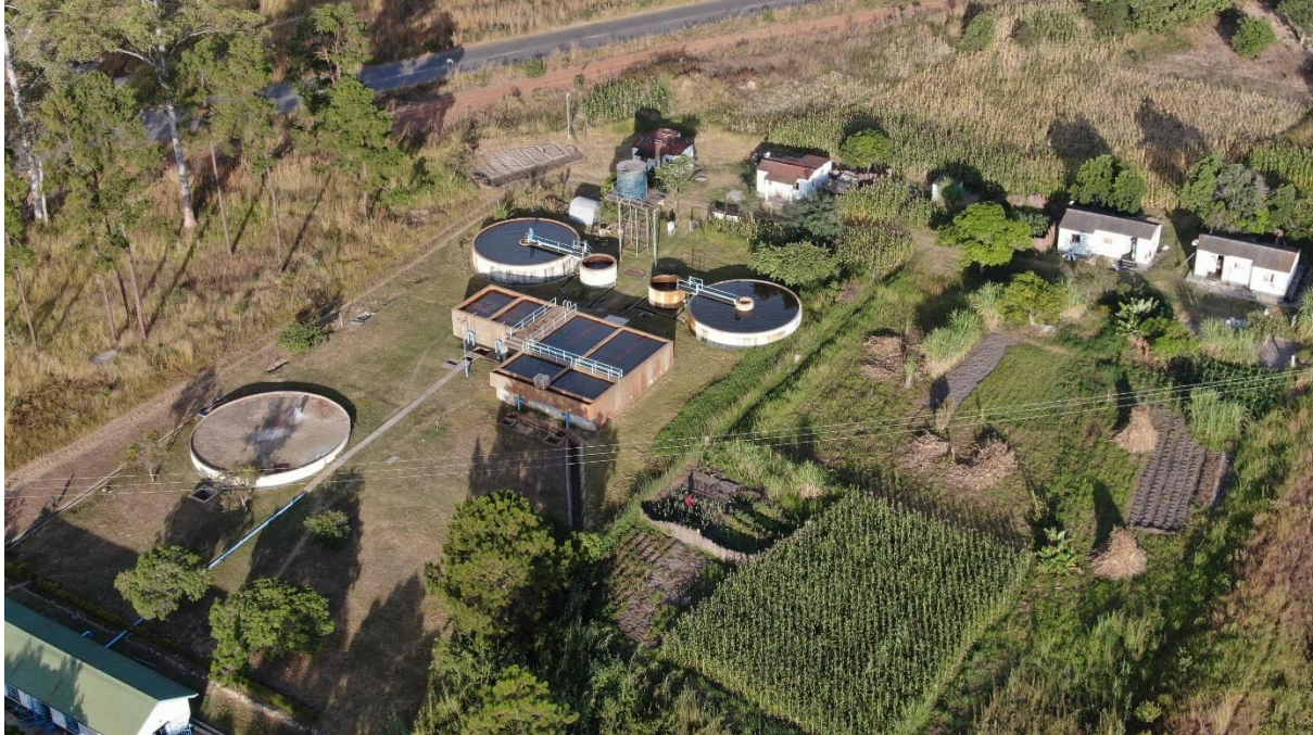
Plate 4.1: Water treatment plant
