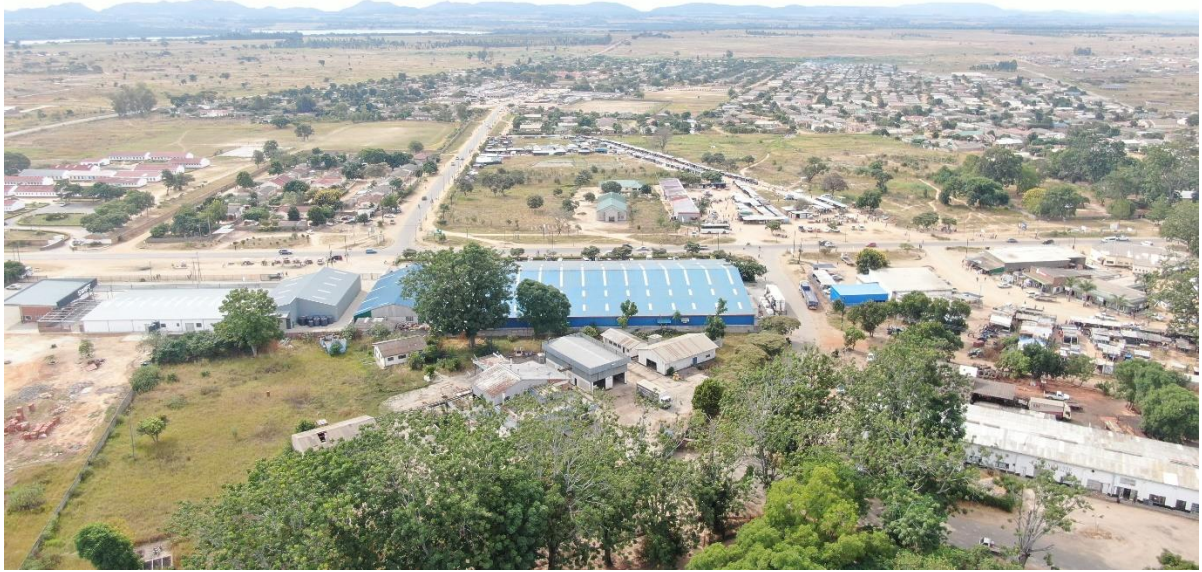
Plate 6.1: Industrial Shells in the Industrial Zone outside the CBD
